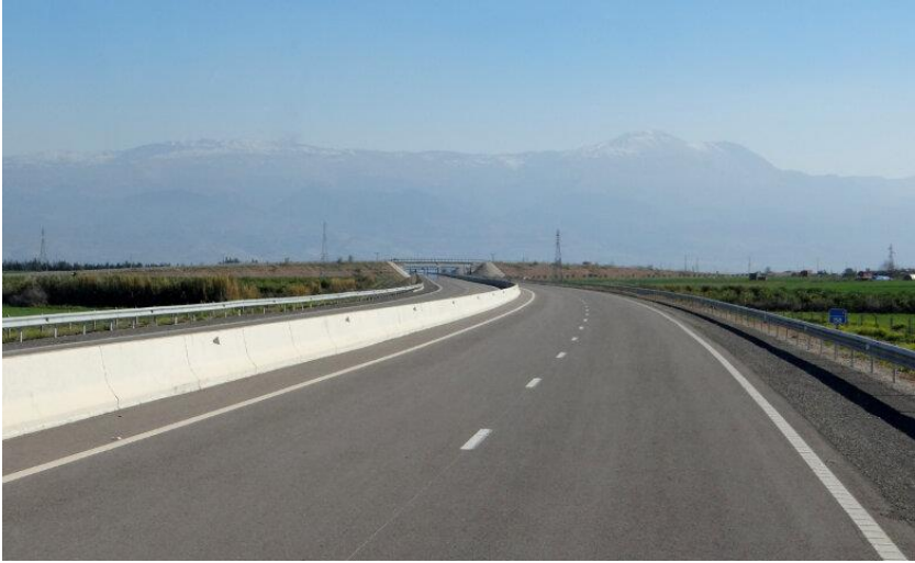
Part of the Moroccan autoroute (motorway) network
